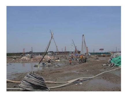
Within the underground area 810 holes with a depth of 92 meters each will be made to place the ground source heat pumps inside of them. The diameter of the U-pipes is 130 mm.
