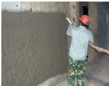
Interior mortar spray
