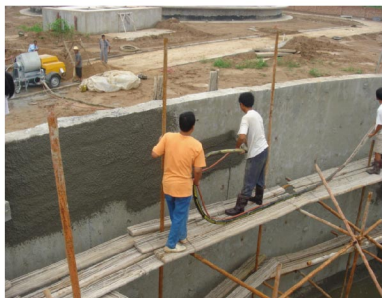
Water Proofing Mortar Spray
