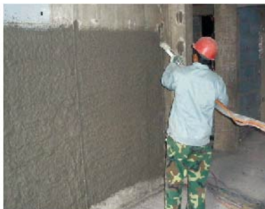
Interior mortar spray
